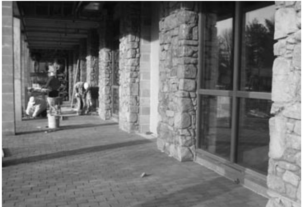
Workers installing brick pavers outside the Smith Education Center's classrooms.
