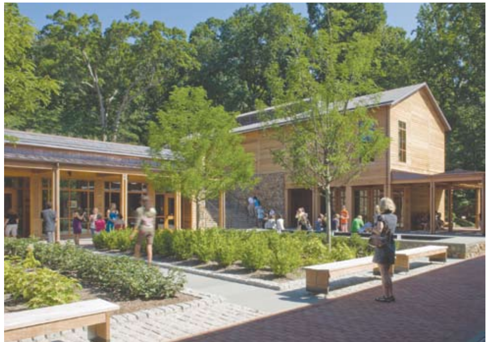
The central courtyard of the Thomas Jefferson Visitor Center and Smith Education Center is one of the facility's two green roofs.
