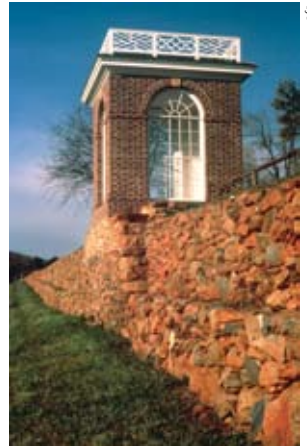
The Vegetable Garden Pavilion atop the restored garden wall.
